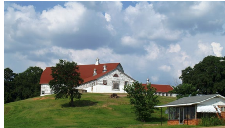
RIGHT RULES, RIGHT PLACE. THE TOOLKIT CONTAINS DIFFERENT RULES FOR URBAN PLACES AND FOR RURAL PLACES. THIS ALLOWS A DIVERSE GROUP OF USERS ARE ABLE TO FIND TOOLS TO BENEFIT THEIR COMMUNITY.
